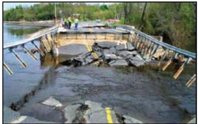
The Rainbow Lake dam was breached, resulting in an 80-ft-long collapse of the entire roadway embankment.
