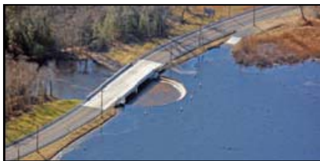
The bridge was designed to accommodate a tangential alignment located on a curved roadway.
